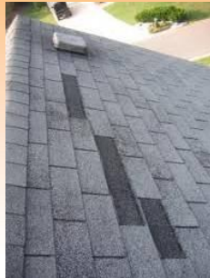
Missing shingle tabs
